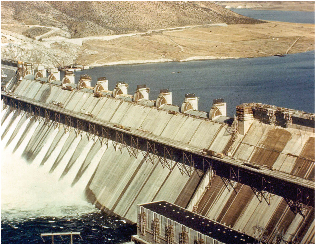
LOOKING EAST OVER THE GRAND COULEE DAM, CIRCA 1941.
