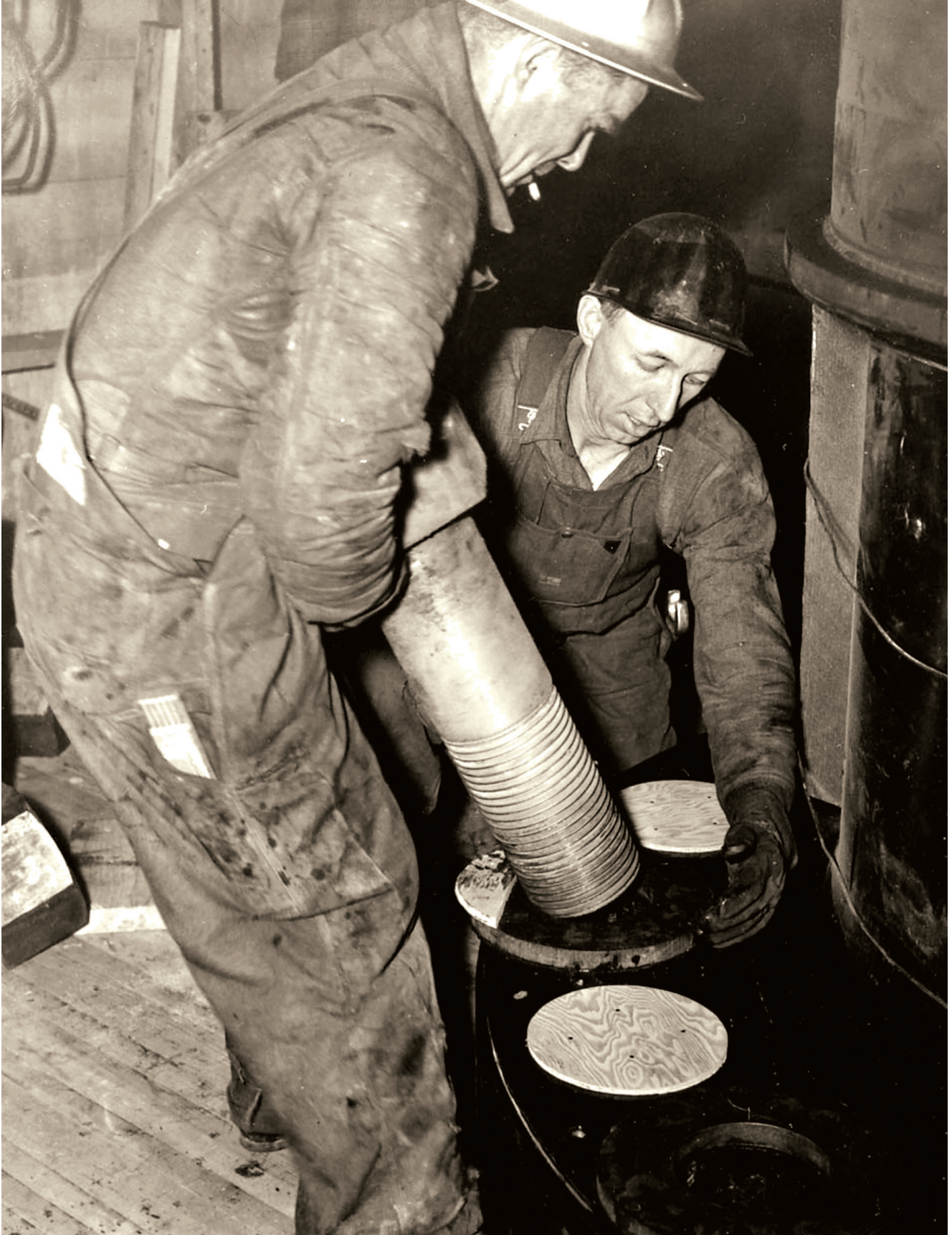
AMOS "TEX" WOOD, STANDING, HELPS POSITION ONE OF THE 120-POUND BOLTS WHICH HOLD THE ROTOR SHAFTS TOGETHER. GRAND COULEE DAM, FEBRUARY 11, 1941.
