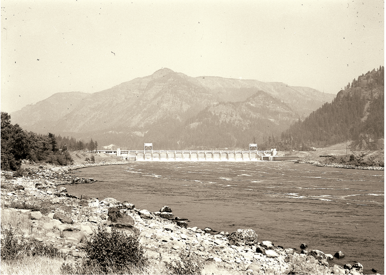
BONNEVILLE DAM DOWNSTREAM, 1940.
