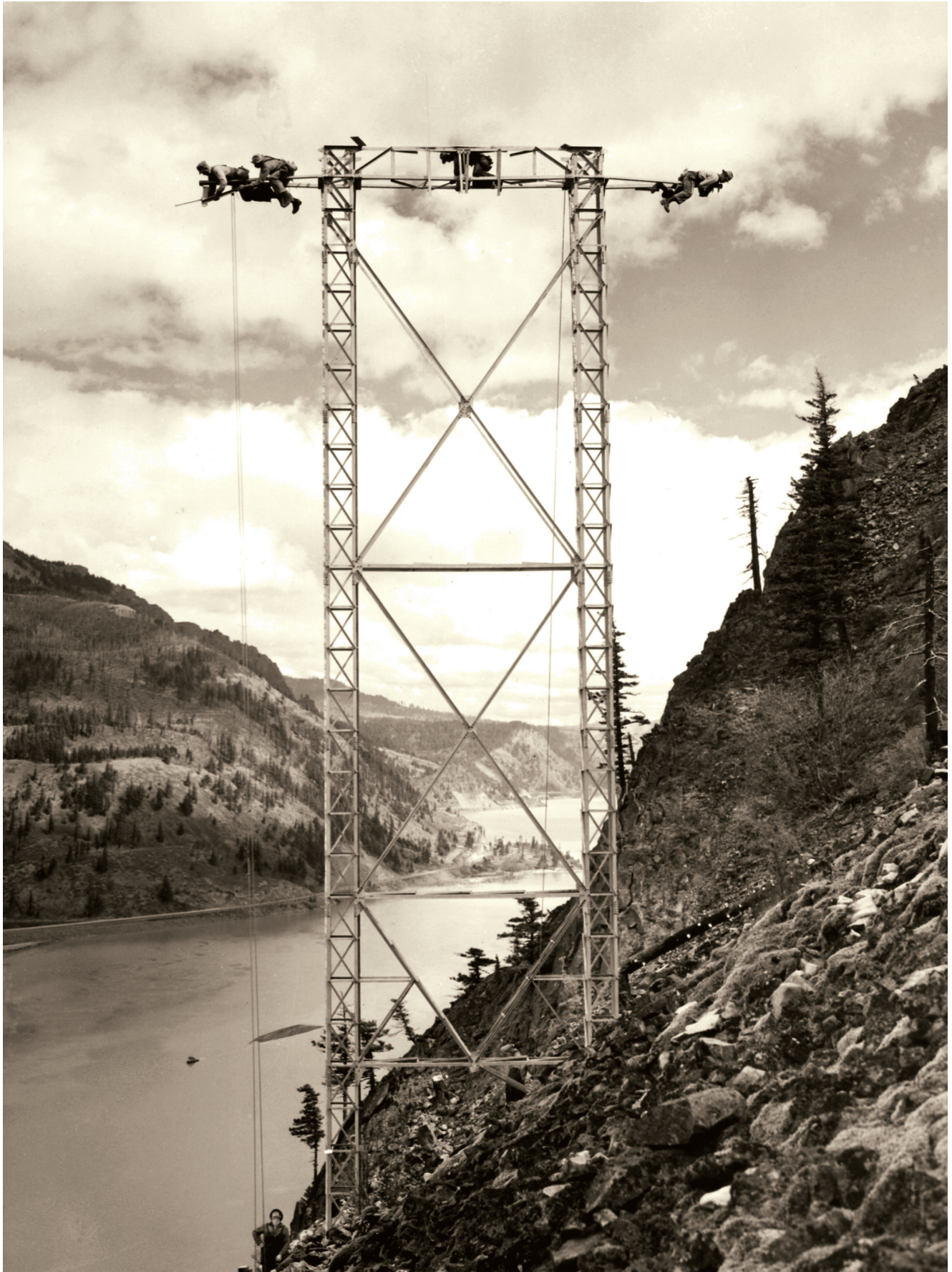
LINE CONSTRUCTION AT THE DALLES, 1941.
